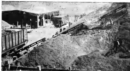
Fig. 2.—Using three Scoop Conveyors to unload from hopper bottom cars to large storage pile.
